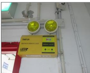
Photo of fire safety equipment Emergency light.JPG
