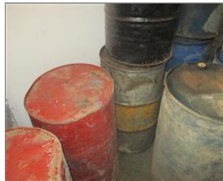
Photo of non-conformity Diesel drums without having secondary containment.JPG
